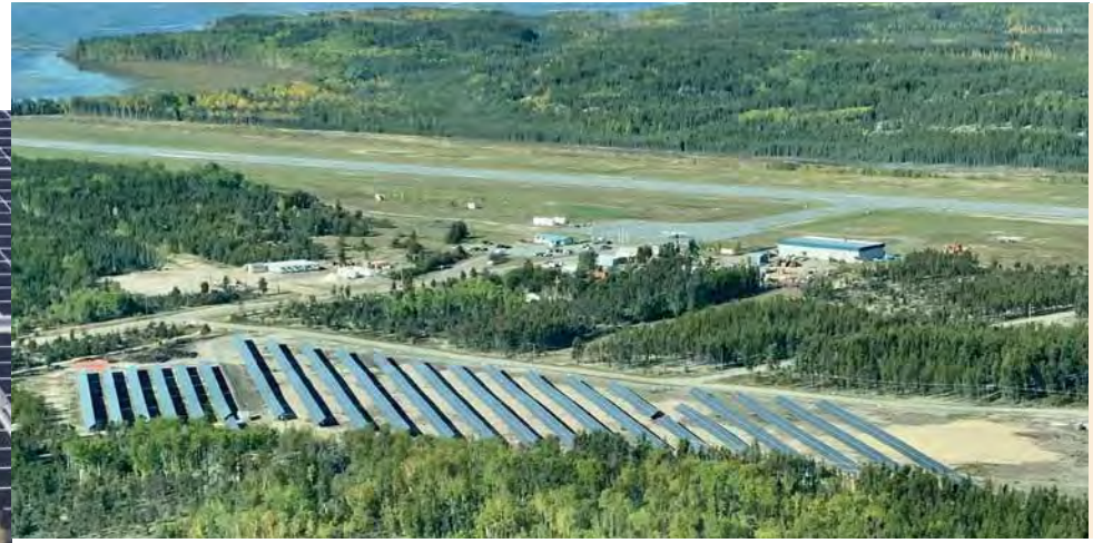
The 2.2 MW solar farm at Fort Chipewyan. The project is owned jointly by the Athabasca Chipewyan and Mikisew Cree First Nations and the Metis Association of Fort Chipewyan. It provides locals with 25 per cent of their electricity needs and reduces the need for diesel.
