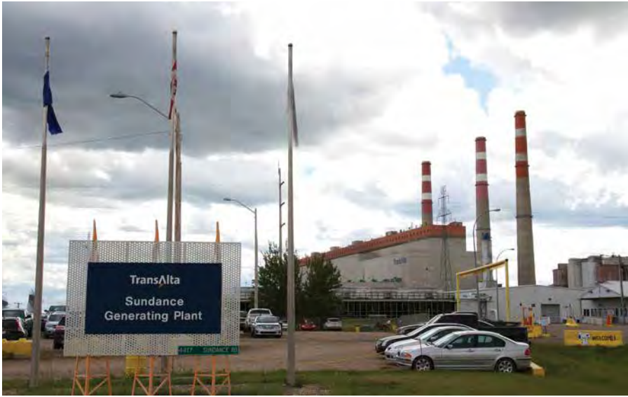
TransAlta's Sundance power generating plant, on Wabamun Lake's south shore, transitioned from coal to natural gas in 2021.
